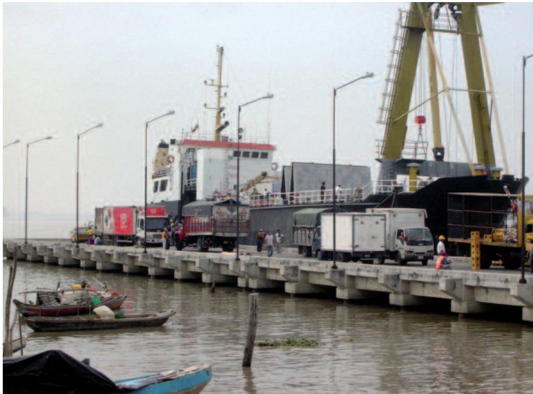
Figure 4. Caraguay Dock in the city of Guayaquil, where cargo ships destined for Galapagos are loaded. There are no mechanical cranes, no areas for pest control, receipt/handling of cargo, or road access to protect food cargo.
